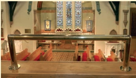
Regularly inspect security of edge protection.
